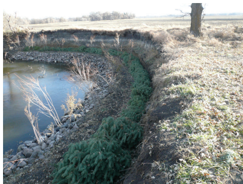
Streambank Stabilization along the Park River. Photo Courtesy of Aaron Sawatzky.
