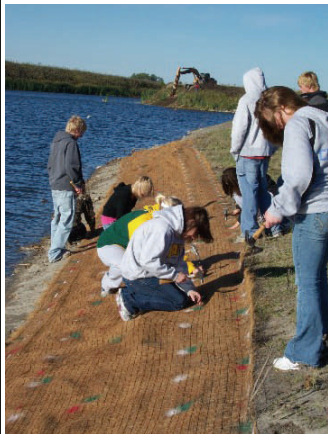
Students installing Erosion Control Blanket.
