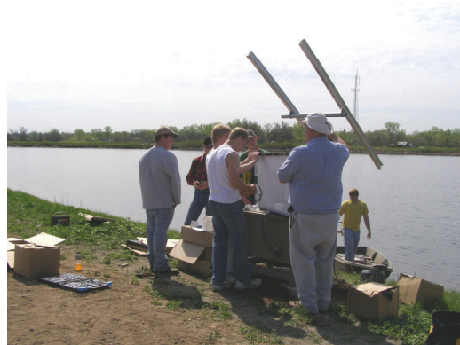
Students and teachers installing the solar powered aeration system.
