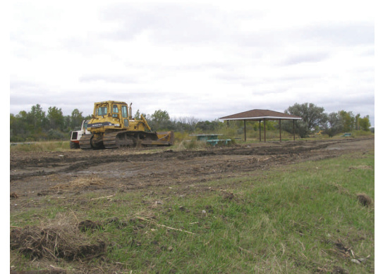
Renovation work was completed by local a contractor.
