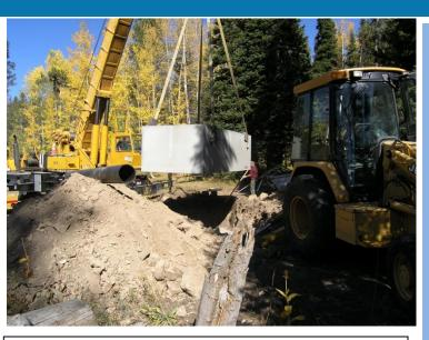
The vault and outhouse were installed on the afternoon of September 30, 2010, by two men utilizing a backhoe to dig a hole for the vault, and a crane to lift the vault and outhouse into place.
