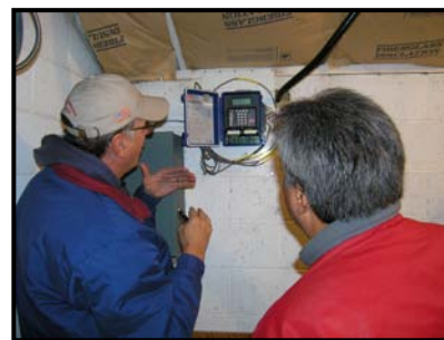
Installation of data logger at Epping, ND tower site.
