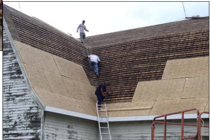
New Roof Under Construction on Prairie Loft Barn (2008)
