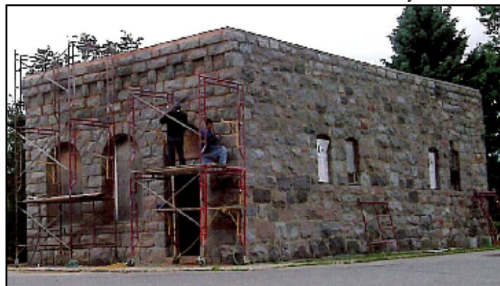
Photo during Restoration
