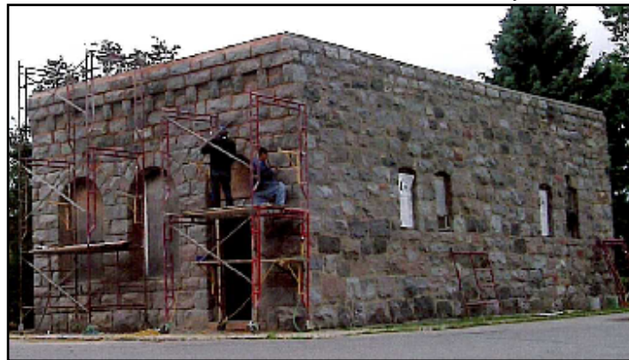
Photo during Restoration
