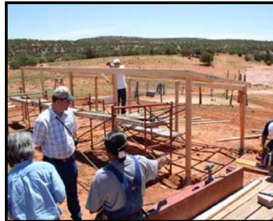
A raincatcher under construction.
